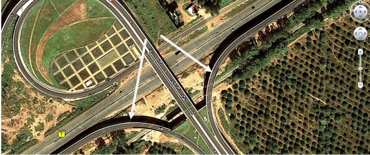
Fig 18: The NH 7 Highway Site
