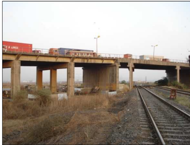
Fig. 3 ROB ( Rail Over Bridge) at Karal Junction, JNPT
