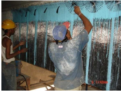
Fig 8 Enclosing the girders with Carbon Fiber Wrapping
