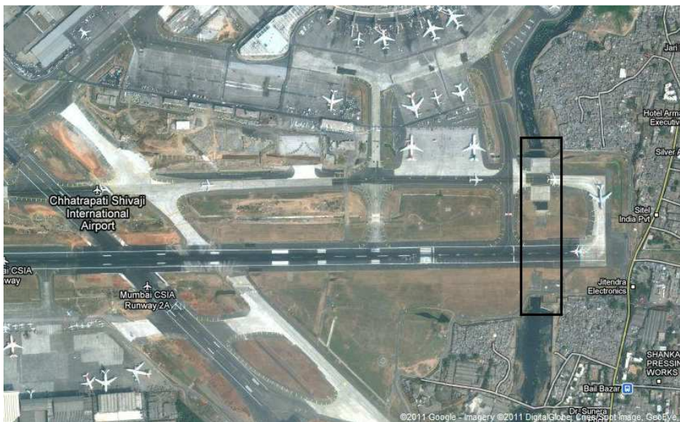
Fig 11 Position of Mithi River Bridge below the runway
