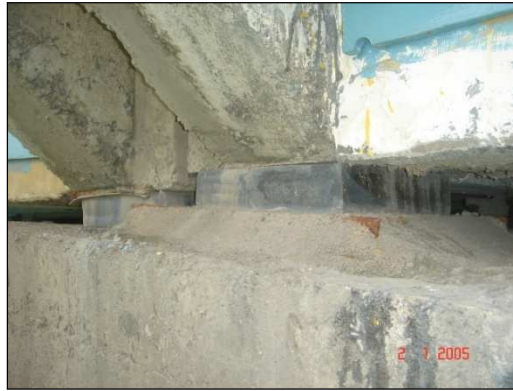
Fig. 6 Replacement of damaged Bearings with new
